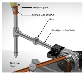
heater factory connections to the gas valve should also be leak tested after placing the water heater in operation.
